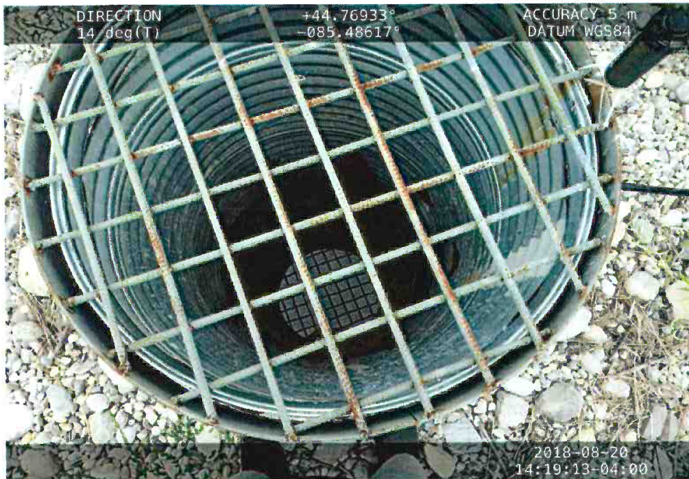
Photo 4: Basin # 1 outflow control structure (exterior)
