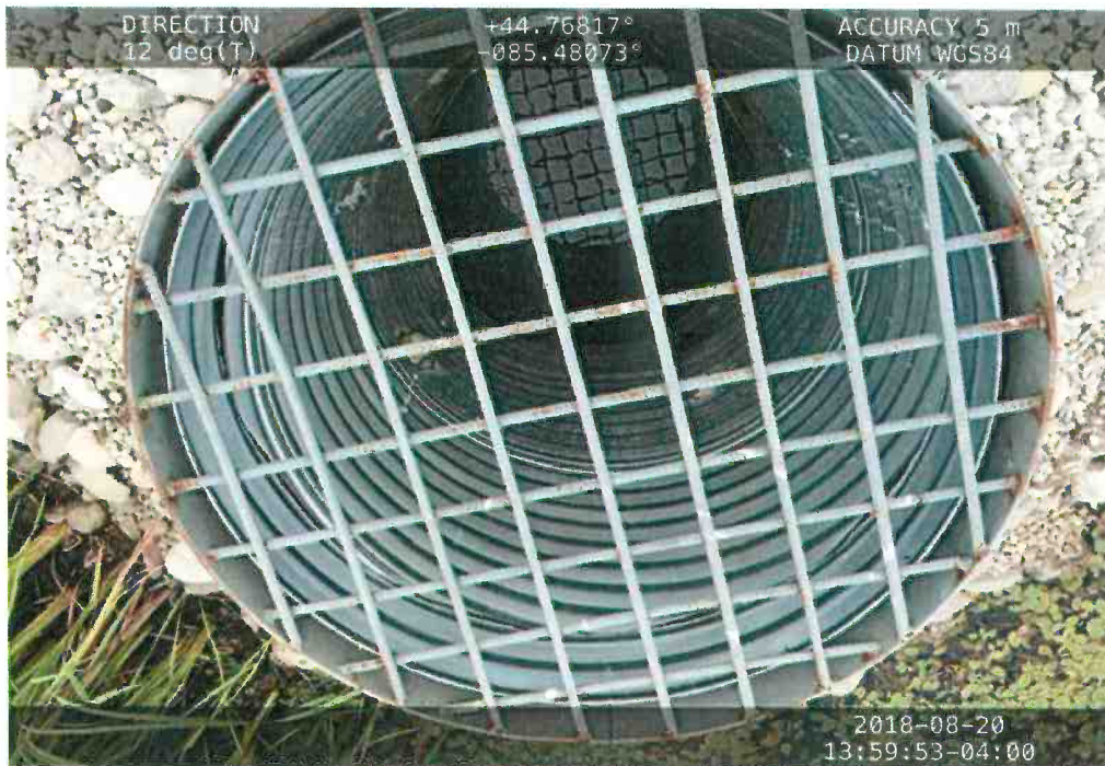
Photo 6: Basin # 2 outflow control structure (exterior)
