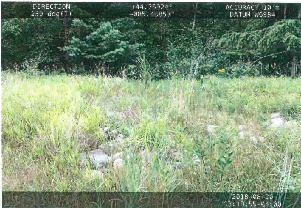
Photo 14: Basin # 2 swale outlet
