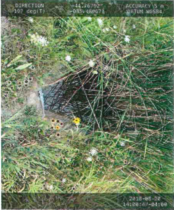
Photo 10: Basin # 1 swale inlet structure
