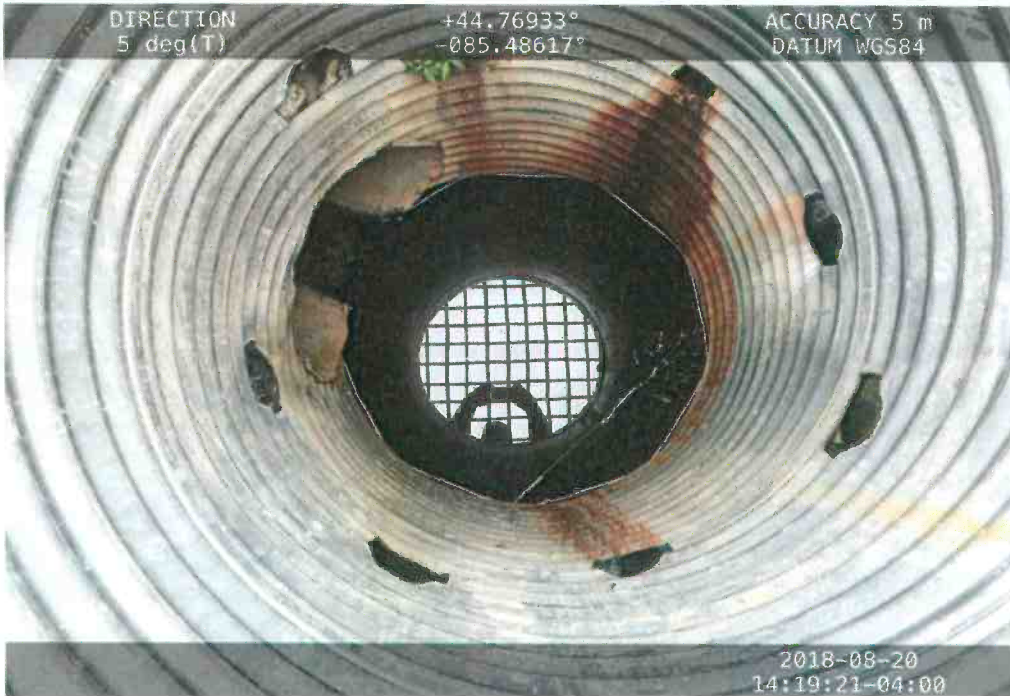
Photo 5: Basin # 1 outflow control structure (interior)
