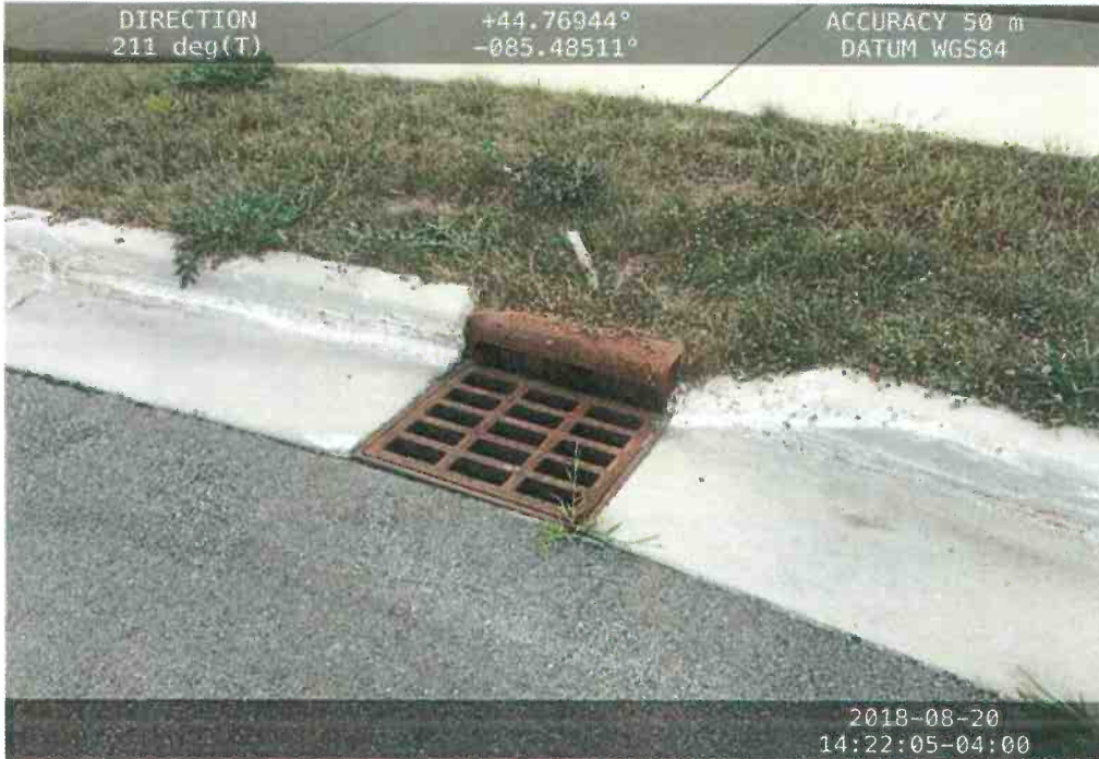
Photo 1: Catch basin inlet west corridor road
