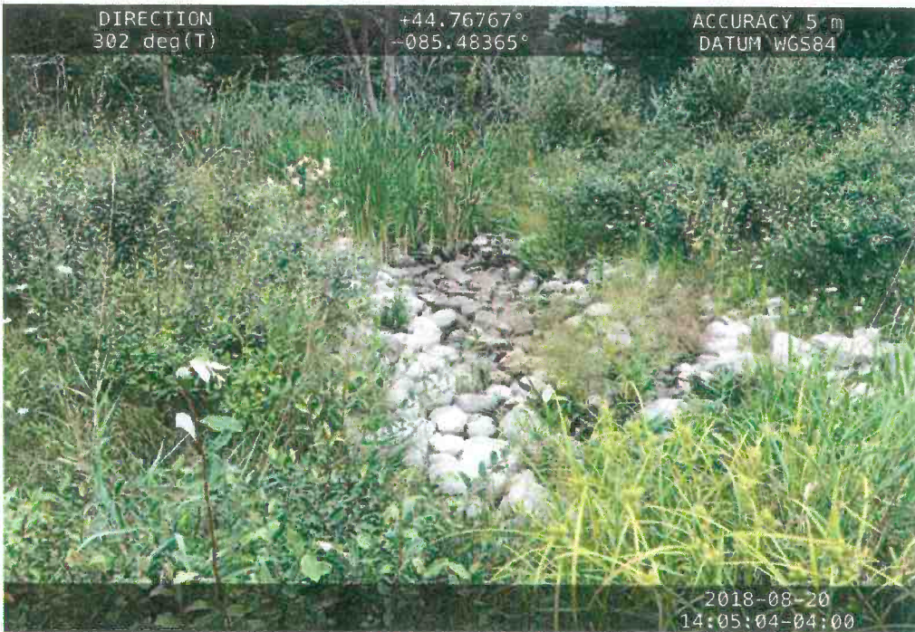
Photo 13: Basin # 1 swale outlet
