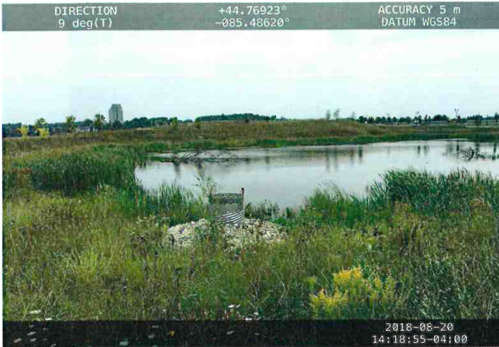
Photo 3: Basin # 2 detention pond viewing north
