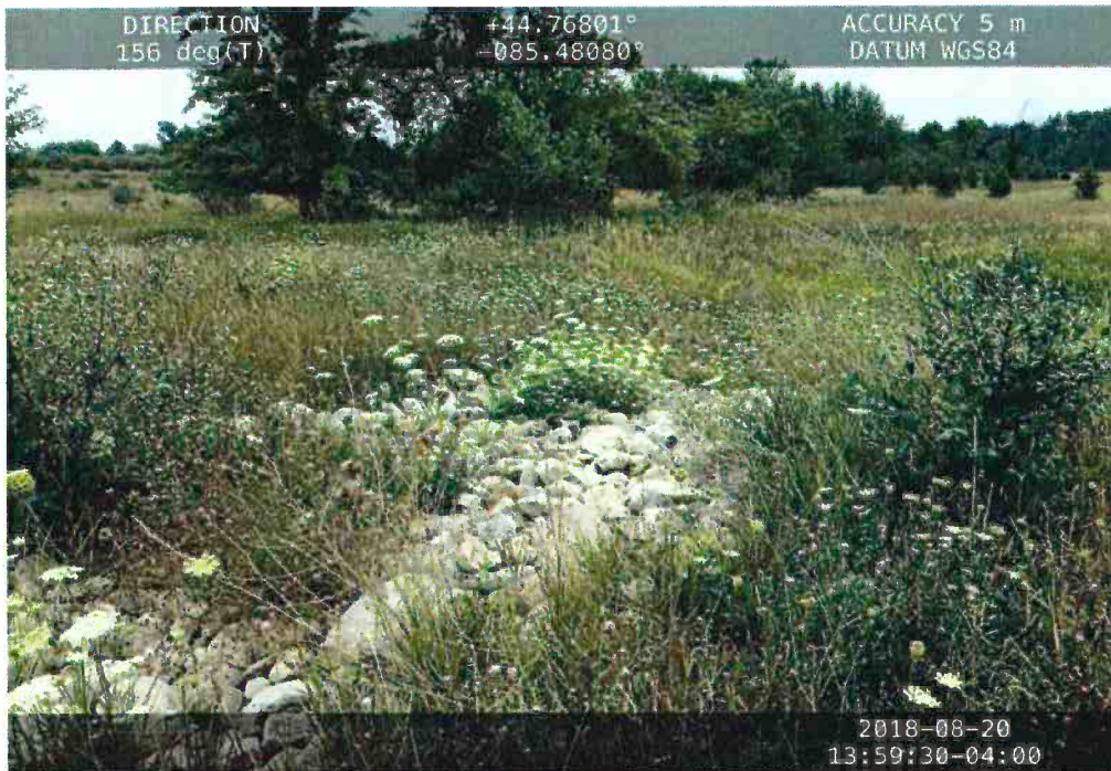
Photo 8: Basin # 1 emergency overflow
